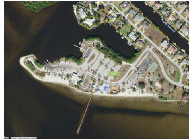
Port Charlotte Beach Complex, 4500 Harbor Blvd, Port Charlotte
