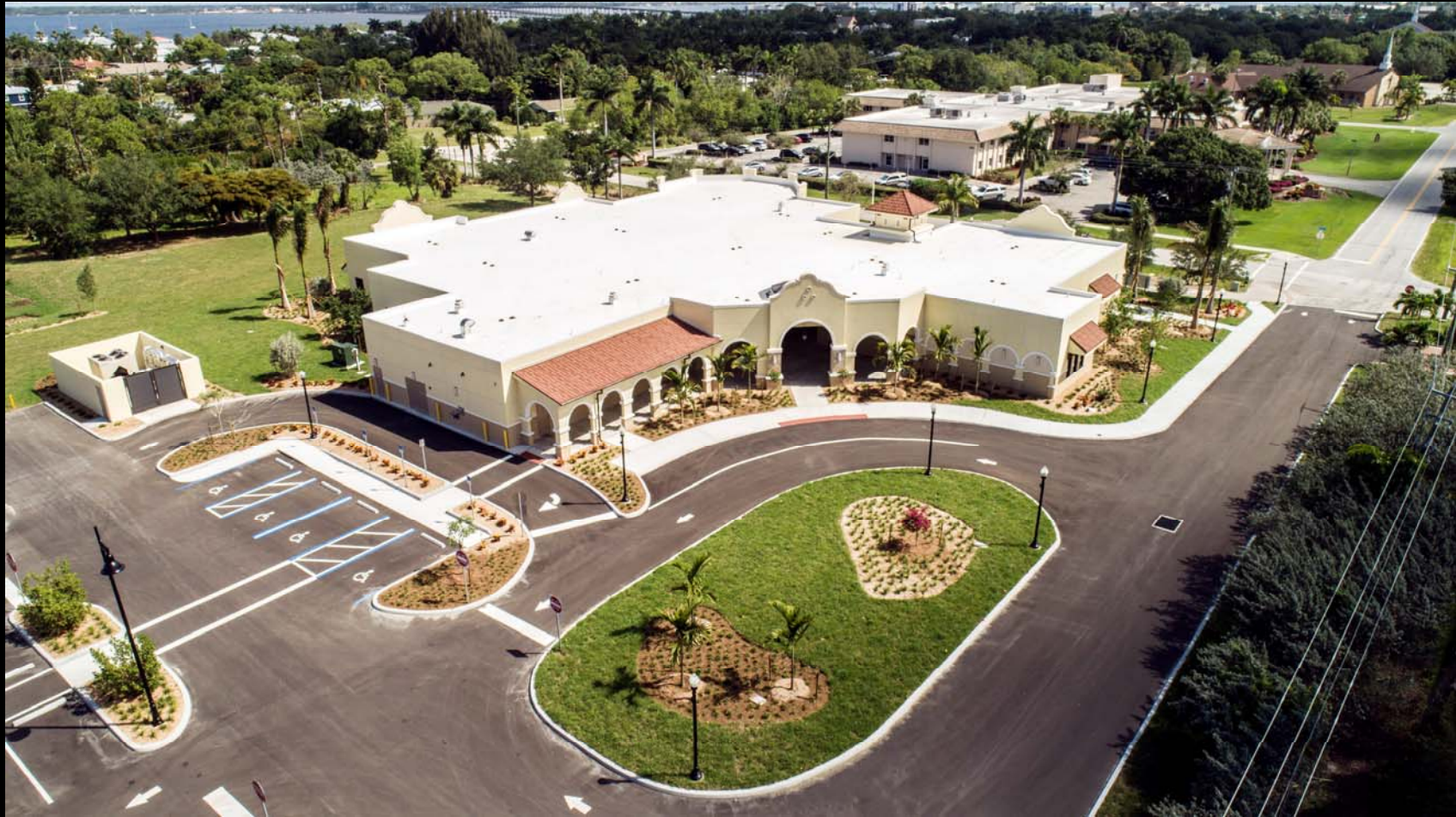
Aerial View from Southwest
