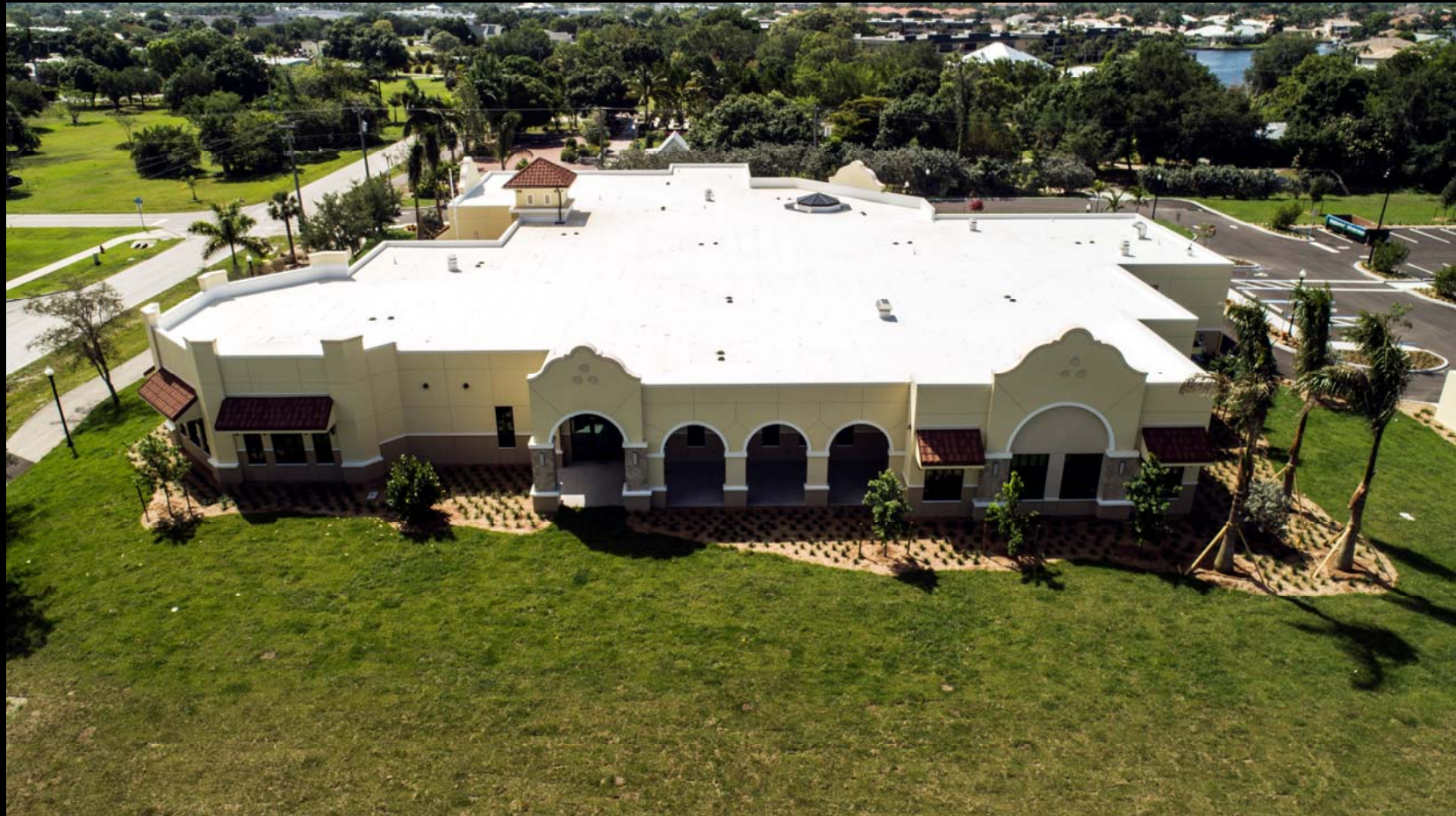
Aerial View from Northeast
