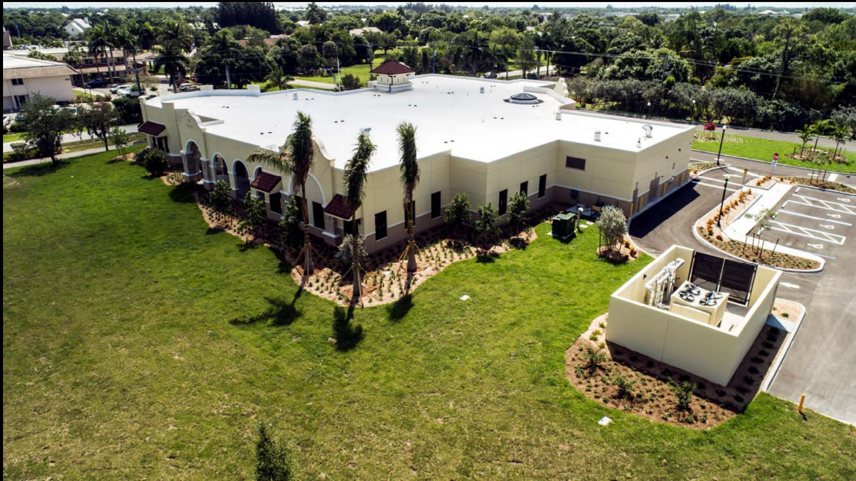
Aerial View from Northwest
