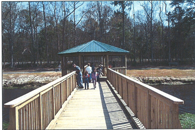
Boardwalk and Gazebo
