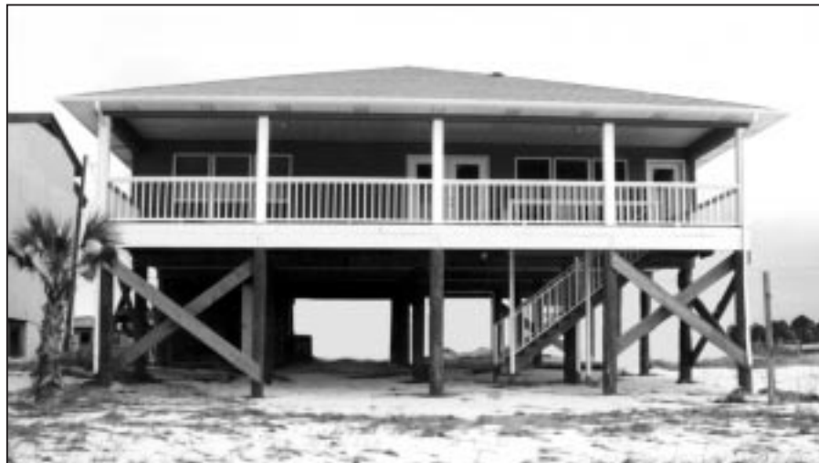
Figure 3-5 This coastal house in Florida was elevated on pilings so that it would be less vulnerable to damage from coastal flooding.
