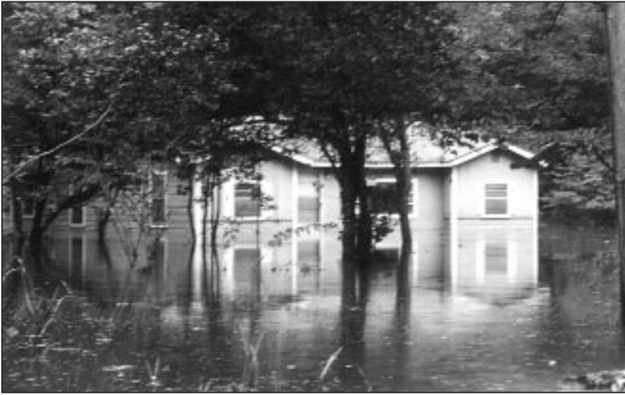
Figure 2-4 This house in Georgia was inundated by riverine flooding.
