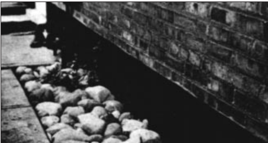
Figure 7-7 a 12-inch-high asphalt coating was added to this brick wall.
