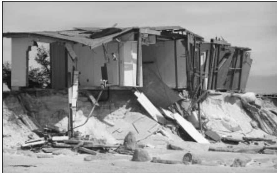
Figure 2-5 The extreme impact of large, fast-moving waves, combined with the removal of supporting soil by erosion and scour, can have devastating effects on buildings exposed to ocean flooding. This house along the Gulf of Mexico shoreline was destroyed during Hurricane Opal.
