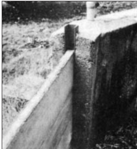
Figure 7-16 Slide-in closure panel.
