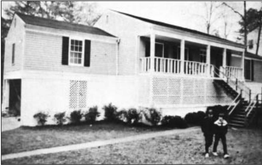
Figure 5-2 This house in Atlanta, Georgia, was elevated one full story. The garage and storage area are at the house's original elevation.
