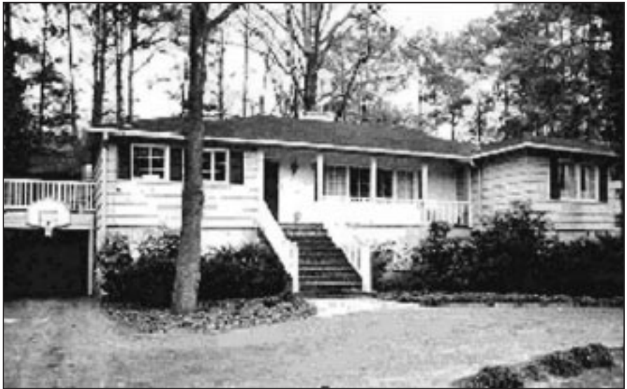
Figure 3-4 Retrofitted house elevated on extended continuous foundation walls.
