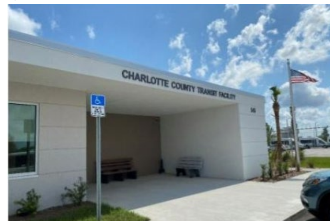
Figure 2-3: CCT Administration and Operations Facility
