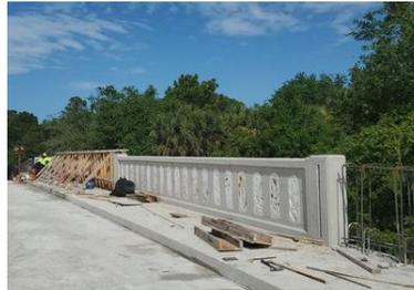
This picture shows the new Texas rail and sidewalk almost complete. The contractor's upcoming work will include curb and gutter, sealing cracks, and roadway work.
