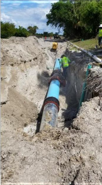
Force mains are pipelines that convey wastewater under pressure from one area to another
