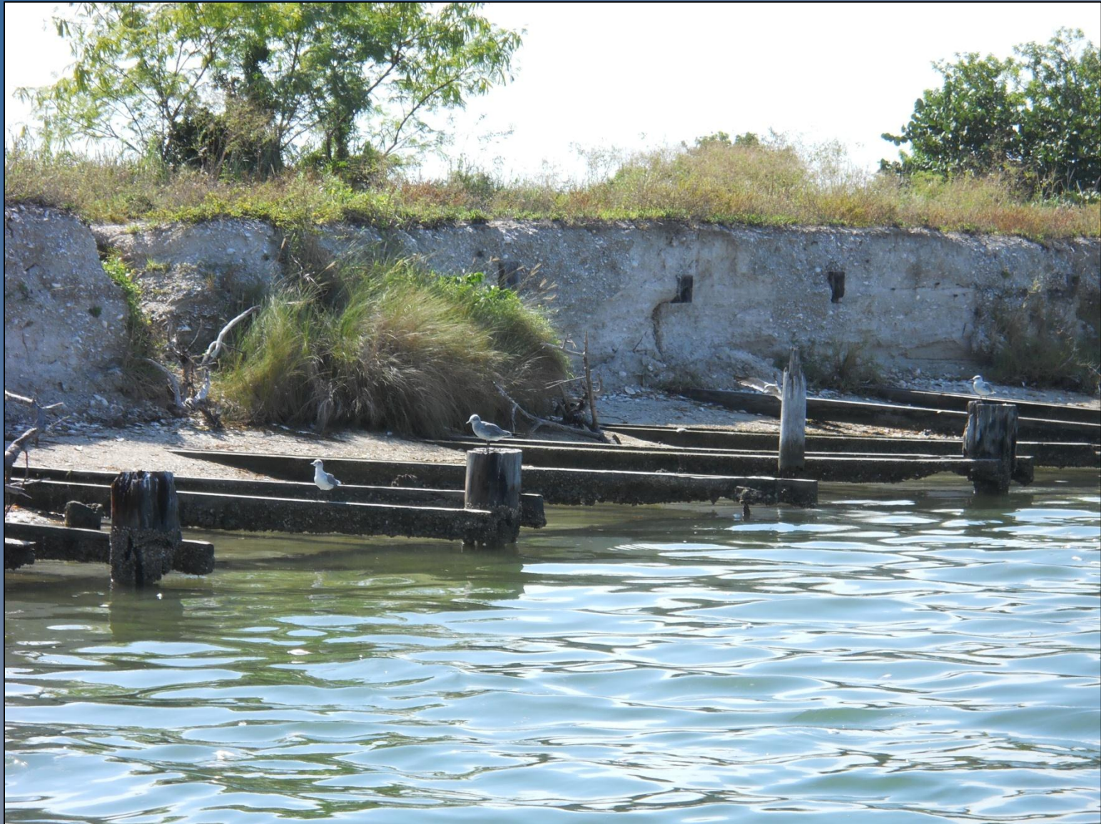
Significant erosion of the soil protecting the trestle along the causeway's spoil island was observed.
