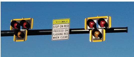
A HAWK (High-Intensity Activated crossWalk) signal is a signal-beacon designed to help pedestrians safely cross busy streets. In 2022 Charlotte County installed a HAWK Signal on Olean Boulevard near Fawcett Hospital.
