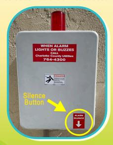
The pump will not function in the event of a power loss. The interceptor tank has a reserve capacity that will allow approximately 8 hours of normal use. excluding washing laundry and bathing, without power. If a power failure occurs, please report the date and time of the failure to the CCU Department.
