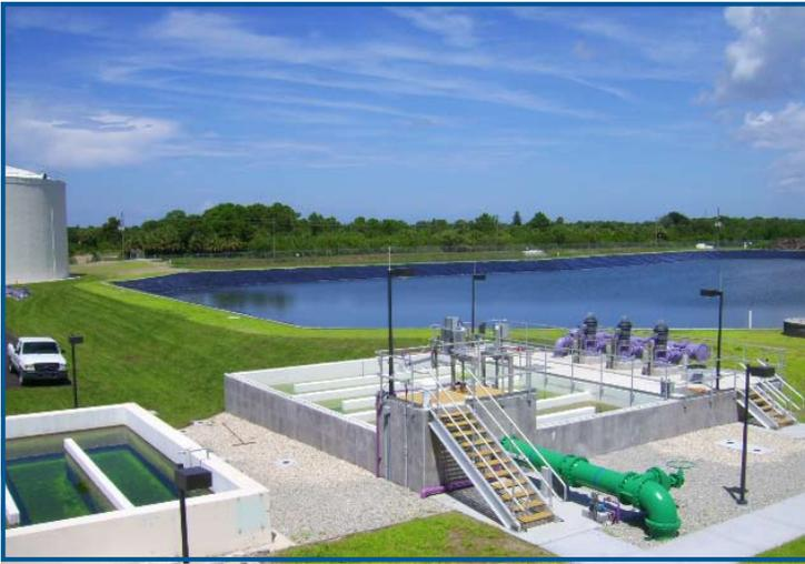
With the improvements complete at the newly renovated Rotonda Water Reclamation Facility (WRF), this facility has expanded to handle 2 million gallons of wastewater each day.
