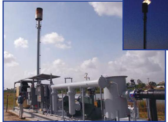
The methane gas-to-energy project at the Zemel Road landfill broke ground in early 2010 and by October Phase I (the flare) was operational. Funded by Mas Energy, the system collects methane the landfill produces and destroys it through a flare (burning) or engines, to be completed in 2011. Both Charlotte County and Mas Energy will receive ongoing revenue from the sale of energy and carbon credits, with the County's portion estimated to be \$800,000 per year.
