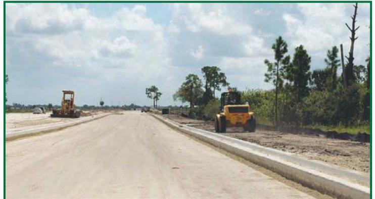
On the Piper Road Project, the curb and gutter is installed before the base material is placed. This step allows for a more efficient work flow, because it is difficult to remove the base material to install the curbing. The curbing also creates a clearly defined space or box for installing the base material in by delineating the road surface and providing a “concrete” (literally) elevation. This material is placed in layers or lifts to ensure that maximum compaction can be achieved.
