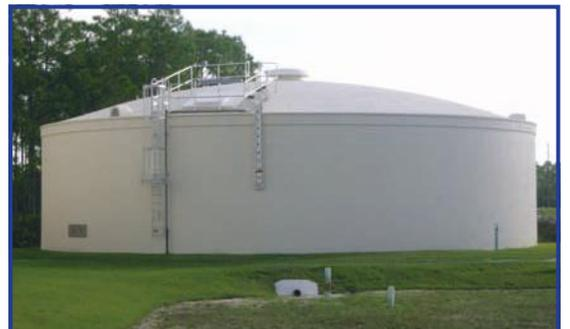
New water storage tanks were part of the expansion of the Burnt Store Water Treatment Plant, completed in 2010. The tanks are capable of holding 500,000 gallons, for the sake of reliability and fire flows.
