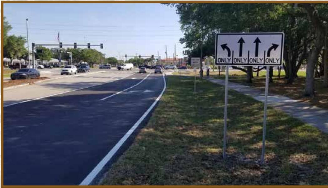
This project consisted of extending the existing right turn lane from Murdock Circle to southbound U.S. 41. The project included new storm drain modifications, construction of the new turn lane along with new signing and pavement markings.
