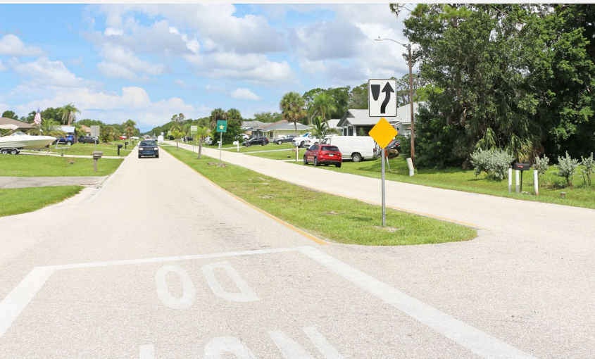
Gillot Blvd. Median East side view
