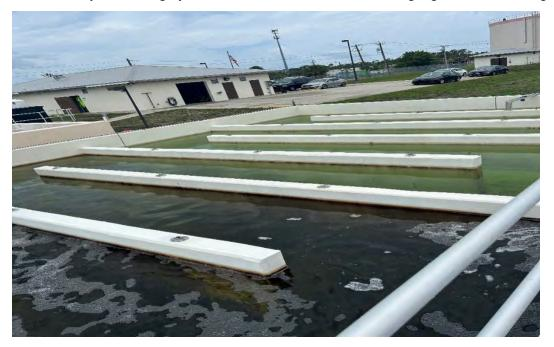
Photo 6: Rotonda WRF Chlorine Contact Basin
