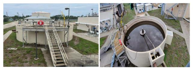
Photo 11: Rotonda WRF Sludge Holding Tanks
