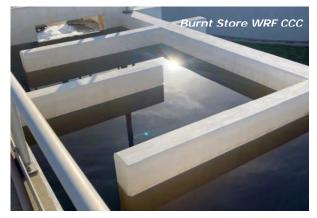
CCC and adjusts the chlorine feed rates. A reagent-less analyzer measures the chlorine residual at the CCC discharge weir for compliance with regulatory limits. Sodium hypochlorite is stored in two tanks with a total capacity of 2,200 gallons.
