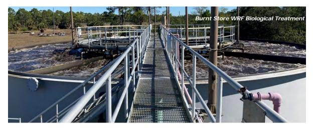
*C. Clarification:* The two steel circular secondary clarifiers are within the center of each package treatment unit for gravity solids separation. The clarifiers are skimmed to remove floatables and scum before clarifier effluent flows over a circumferential weir to the tertiary filters.
