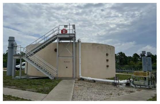
Photo 1: Rotonda WRF Flow EQ Tank
