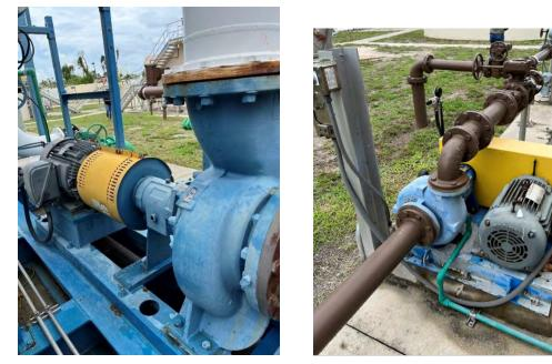
Photo 12: Rotonda WRF RAS Pump Photo 13: Rotonda WRF WAS Pump
