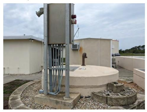
Photo 14: Rotonda WRF Plant Drain Collection and Pumping System
