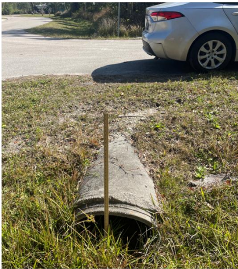
Figure 4: Site visit photo of typical Tropical Gulf Acres pipe crossing
